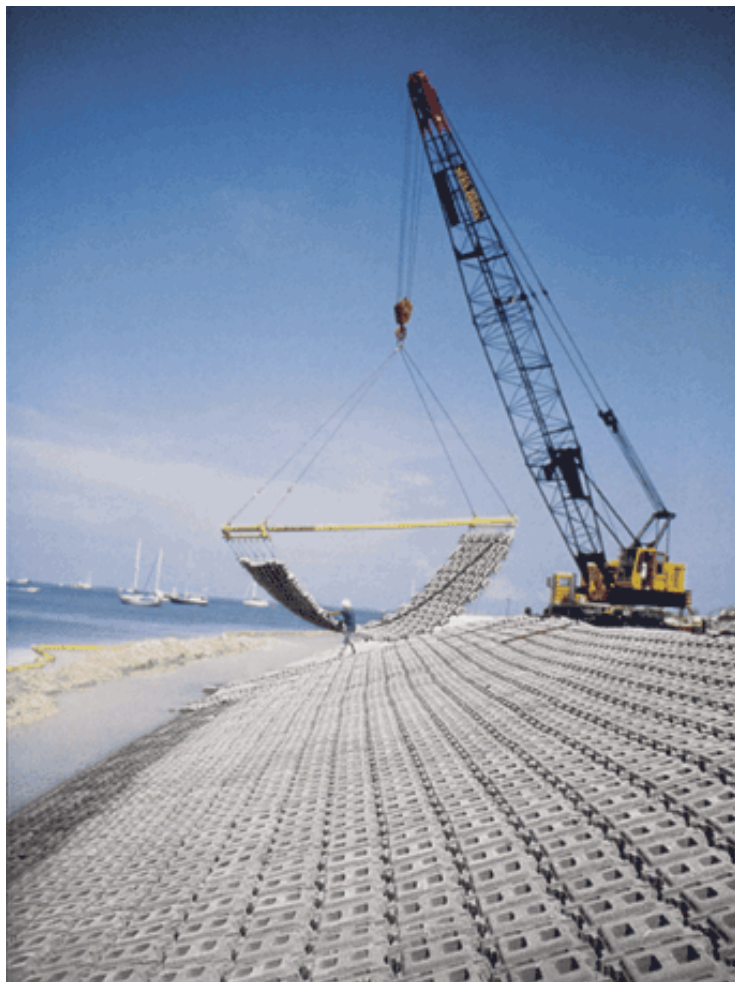
Figure 5—Placement of Cable ACB System With Crane
