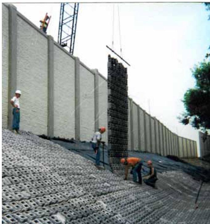
Figure 6—Cabled ACB Installation Behind a Sound Barrier
