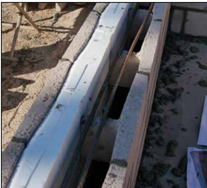
Hi-R H units are suitable for construction of bond beams without the need for any modifications to the units and the insulation inserts remain fully in place
