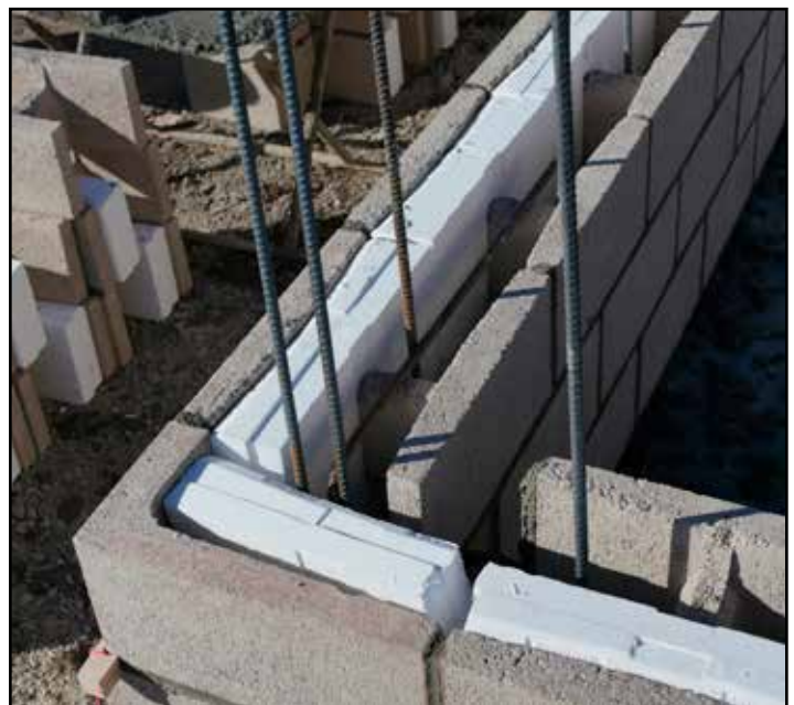
Insulated corners are built using conventional masonry fittings and Hi-R H units
